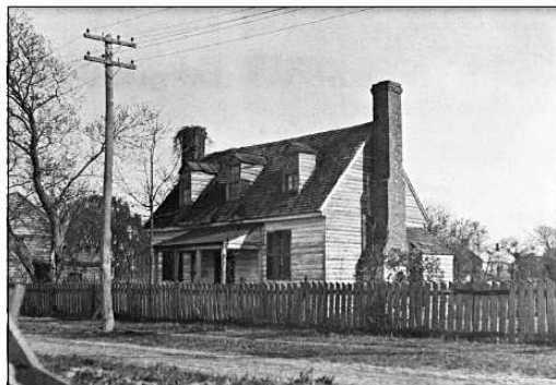
Front elevation of the Dudley Digges House/Bray School in its original location on Prince George Street, Williamsburg, Va. Earl Gregg Swem photo, 1921. Courtesy Special Collections, John D. Rockefeller Jr Library, The Colonial Williamsburg Foundation.
