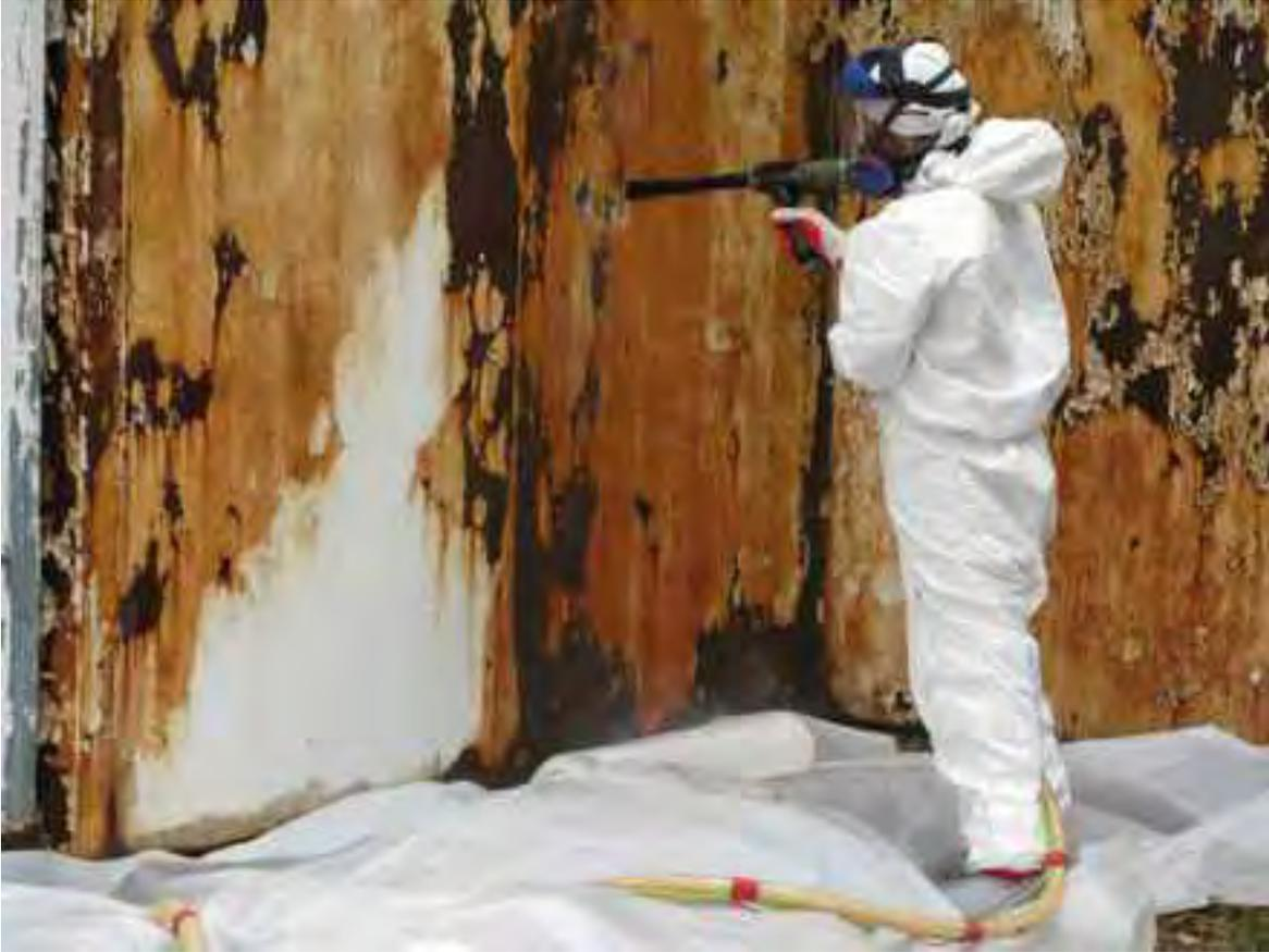
**Workers from Yankee Fiber Control Inc. employ dry ice blasting to remediate lead-based paint at the steel house in March 2009 (author photo)**
