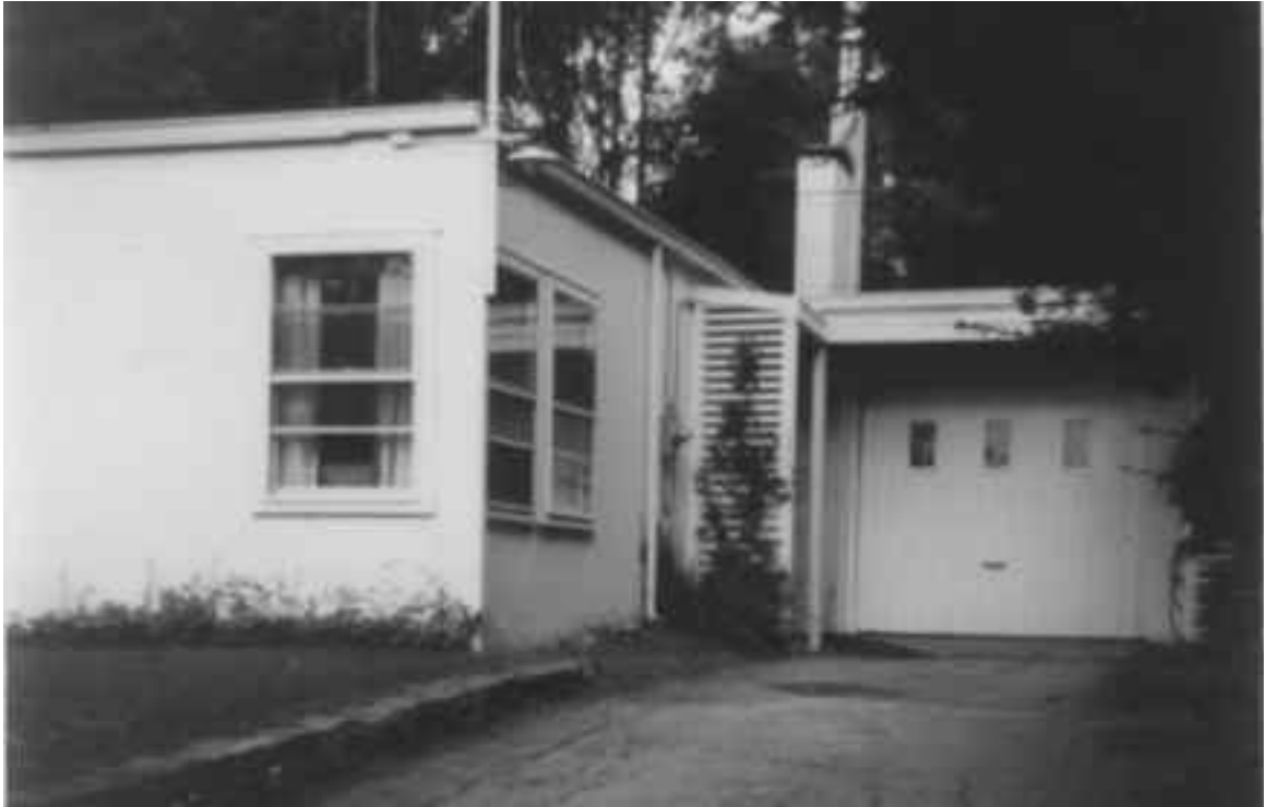
Connecticut College reference librarian Jim MacDonald’s snapshots show the steel house in the early 1970s, about a decade before the pitched roof was added (photo: James MacDonald)
