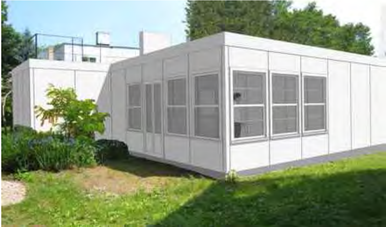
Rendering of a rehabilitated steel house as conceived by Barun Basu Associates, the project’s preservation architects, in 2010 (photo illustration by James Dixon/Barun Basu Associates)
