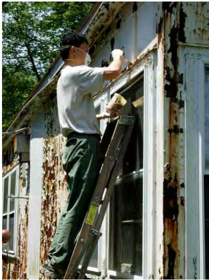
Connecticut College professor Tek-wah King, a former resident of the steel house, “paints” the building with calcium sulfonate penetrant in 2008 (left); a coating of rust is visible behind peeling paint (author photos)
