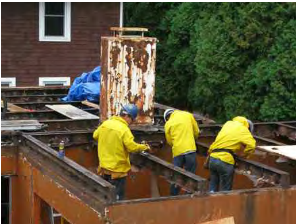
Milner + Carr conservationists “unbuckle” U-shaped steel roofing members in the steel house’s attached garage, September 2011 (author photo)
