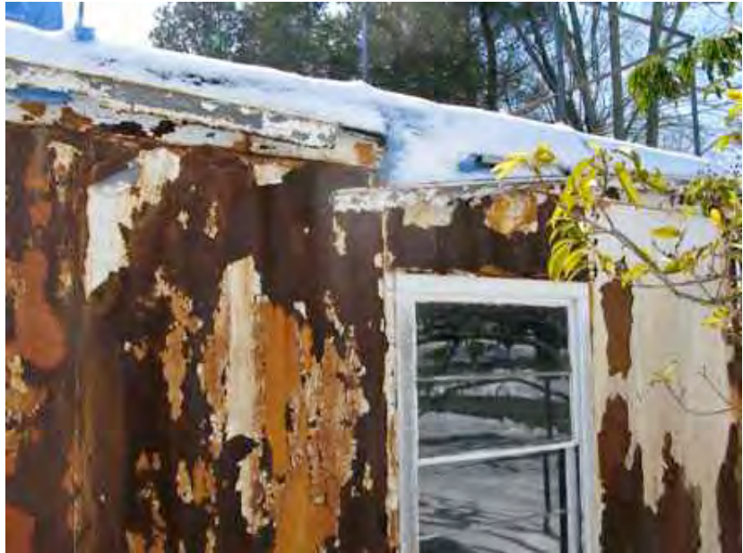
Connecticut College professor Tek-wah King, a former resident of the steel house, “paints” the building with calcium sulfonate penetrant in 2008 (left); a coating of rust is visible behind peeling paint (author photos)
