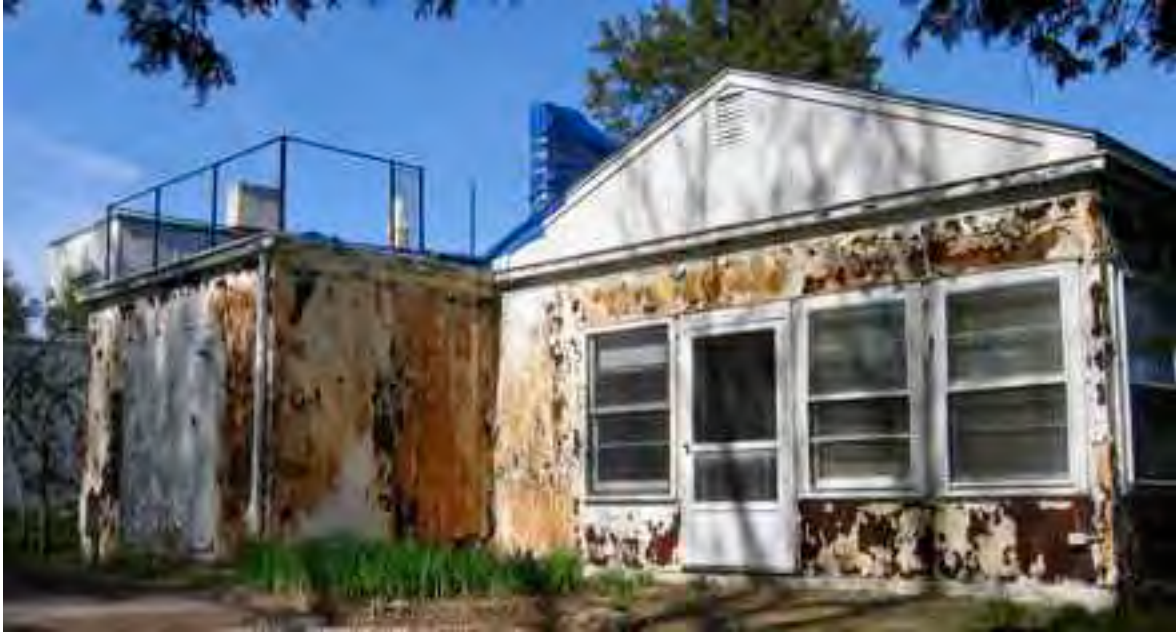
In 2007, Connecticut College's steel house, designed and built by General Houses, Inc., in 1933, stood vacant and in disrepair (author photo)
