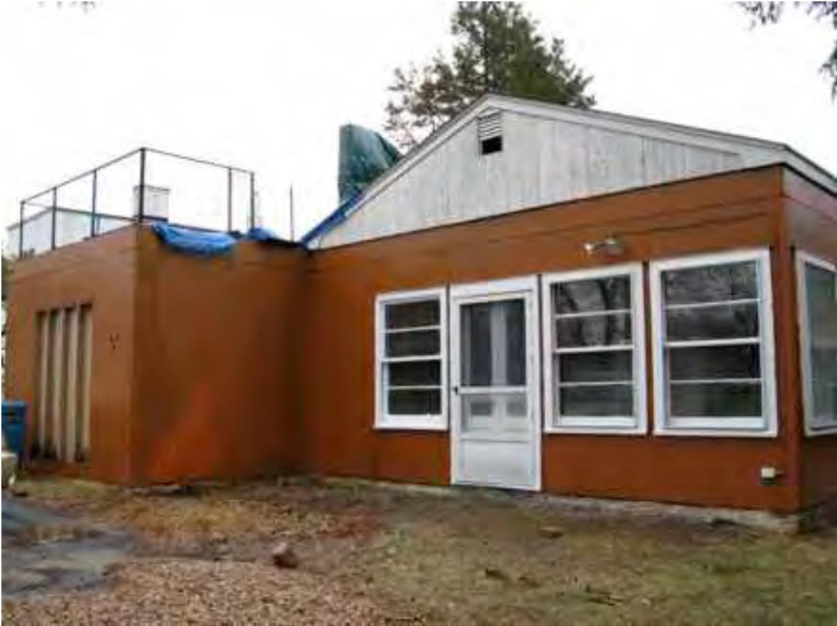
**The steel house after Yankee Fiber Control had abated the peeling lead-based paint and applied Prax-Ten Penetrant to bare steel surfaces in April 2009 (author photo)**
